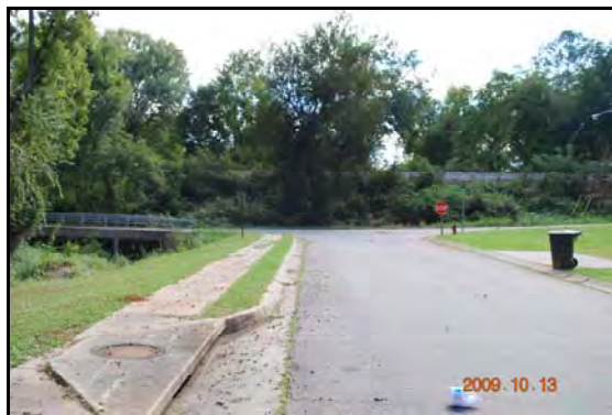
Figure 26: Southeasterly View Down N. Liberty Street Toward Railroad Track
