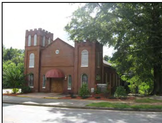
Figure 21: Double Tower Church (ECA #38)
