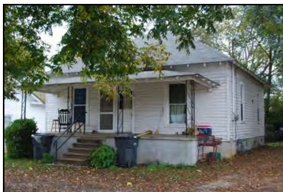
Figure 14: Central Hall Cottage (ECA #147)
